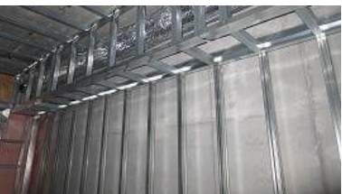
Metal (for plasterboard base: light steel frame)
